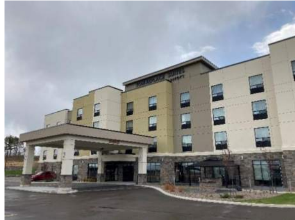
Figure 3-11 Example of building façade on new construction (Source - WSP)
