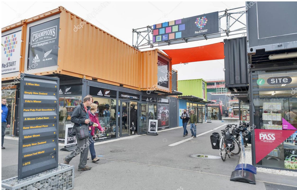
REstart – Christchurch, NZ SECOND LEVEL CONTAINERS, THE GLAZING AND SOLID WALLS PLUS THE DISTANCE BETWEEN CONTAINERS CREATE A STREET SCALE SENSE OF ENCLOSURE
