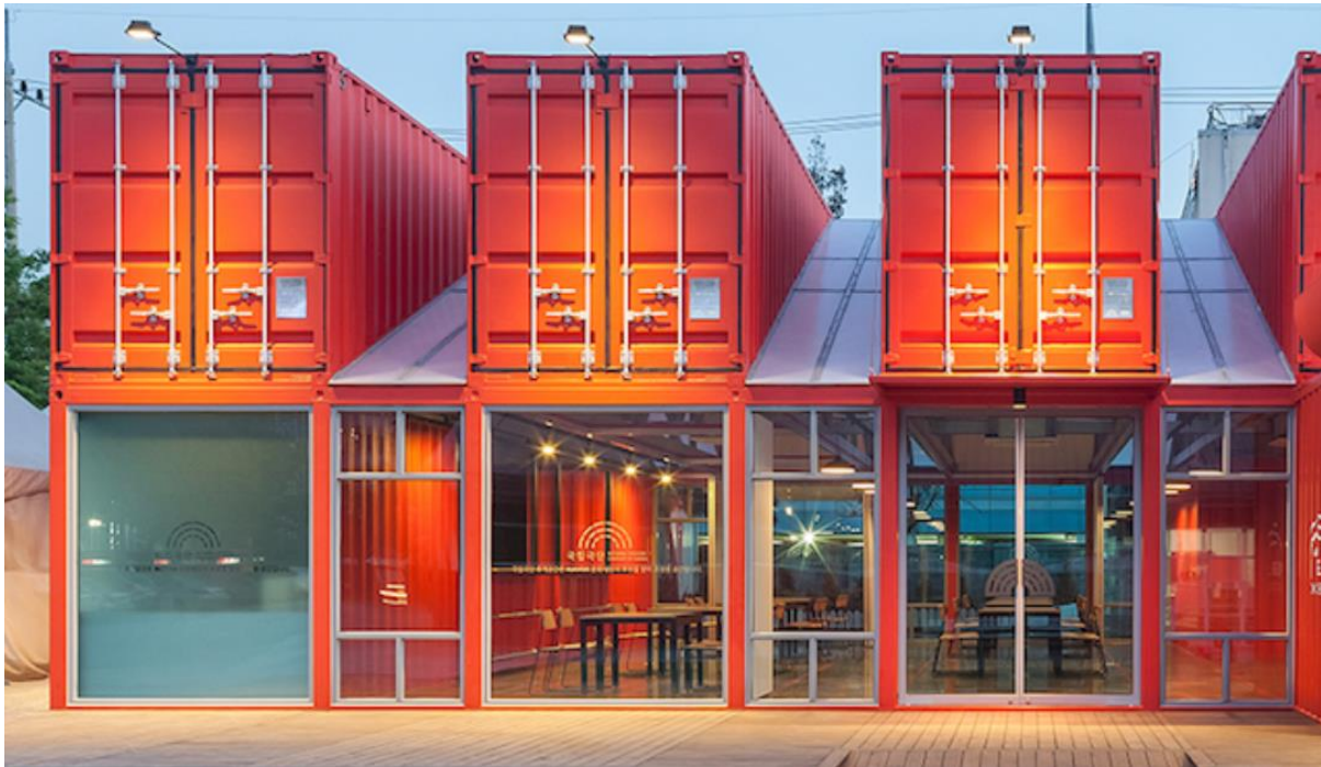
Korea – Inhabitat.com TRADITIONAL STREET SCALE PROVIDED THROUGH STORE FRONT GLAZING AND SECOND LEVEL CONTAINERS.
