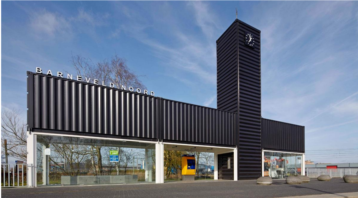
Germany STREET SCALE PROVIDED THROUGH STORE FRONT GLAZING AND SECOND LEVEL CONTAINERS. VERTICAL CONTAINER LANDMARKS THE PROJECT. — ARCHDAILY.COM
