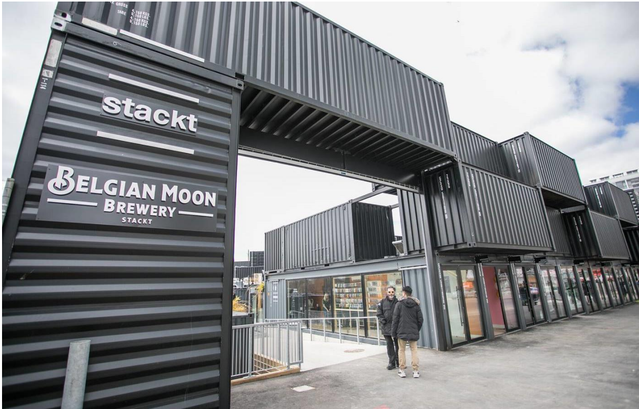
Stackts, Toronto, DEVELOPMENT ENTRANCE DEFINED BY CREATING AN ARCH WITH A SECOND LEVEL CONTAINER.
