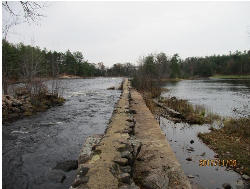
Rock Wall (Looking East towards the Island)
