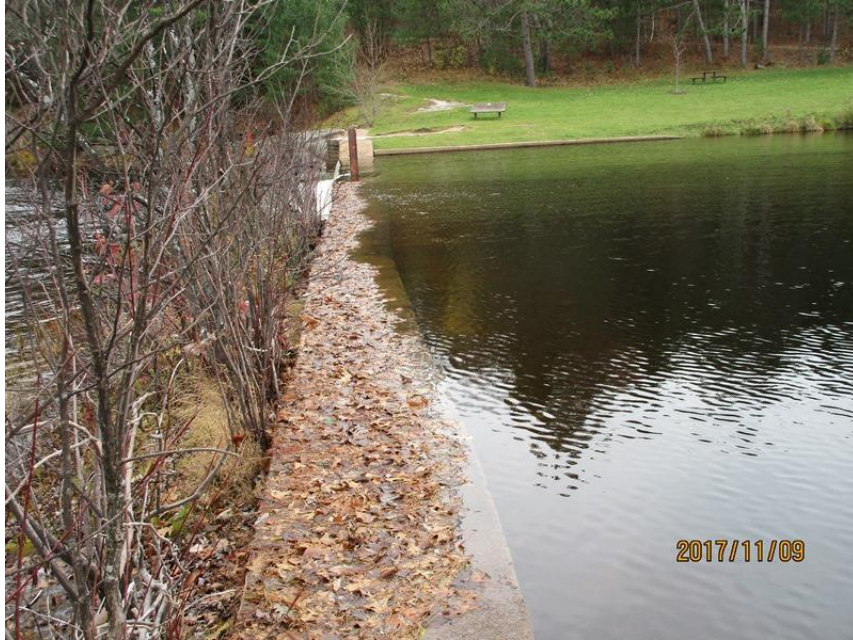
Outflow Wall – Looking South East (overtopping taken from Island)
